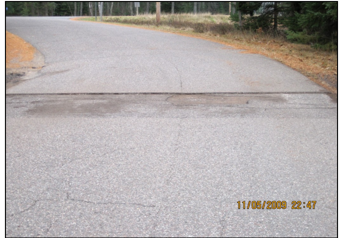
Butt Joint Milled for Smooth Transition Prior to Resurfacing
