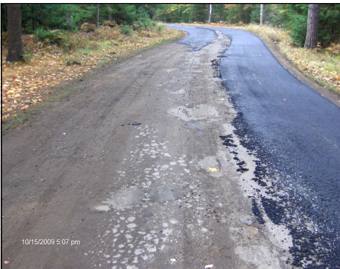
Safar Road/Three Lakes - Wedge Layer Prior to Resurfacing
