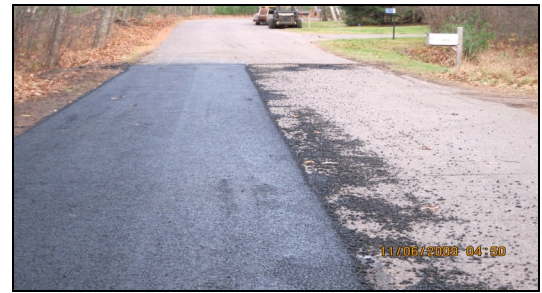
Photo of New Road Hot Mix Asphalt construction
